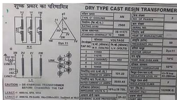
Gambar 7 Name Plate Transformator
